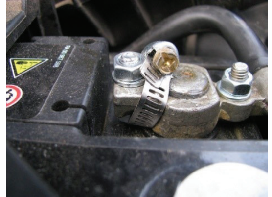
Temporary Hose Clamp Repair
